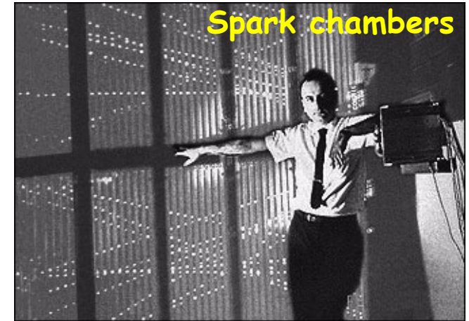
Sandwich of Aluminium plates and spark chambers
