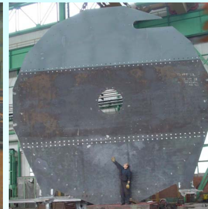
Large steel plates were manufactured in Serbia.
