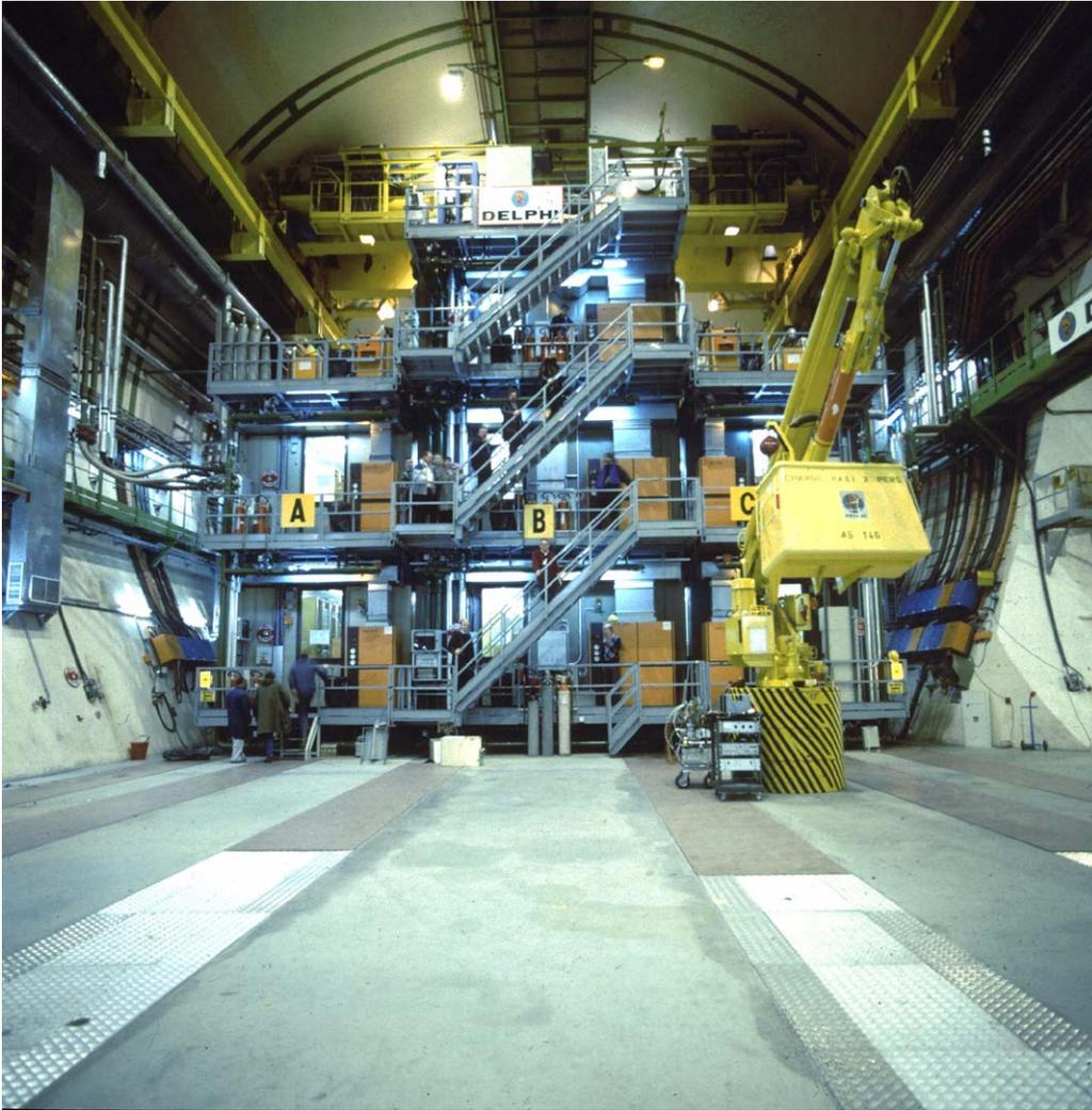
The photo shows the DELPHI cavern with the buildings for the electronics hiding the experiment.
