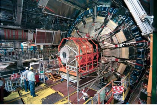
Figure 3. The insertion of the SCT and the TRT Barrel in the Barrel Calorimeter.
